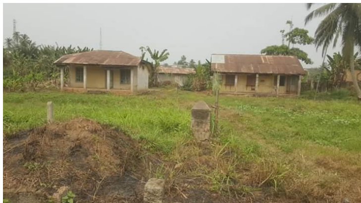
Figure 1 2018 view of Ejinrin Post Office (right) and Postmaster's house (left)
